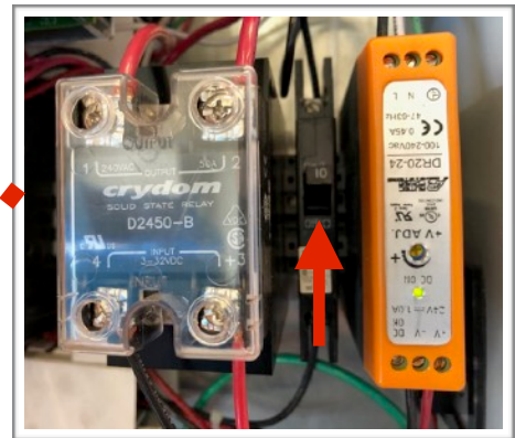
1) AC power controlled by circuit breaker
